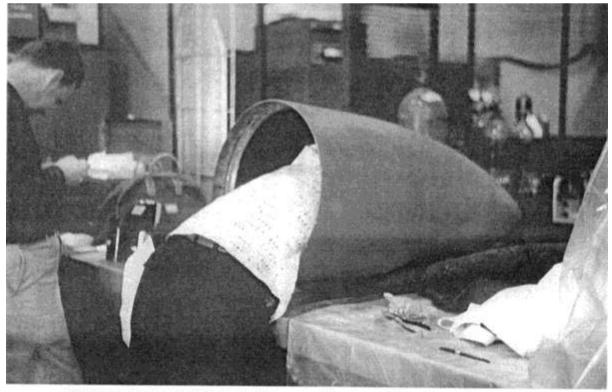
1961: Goddard Space Flight Center: installing a parasitic antenna inside a heat-resistant nose cone.
