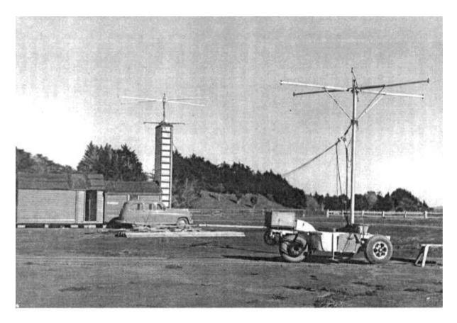
1953: MUCH WINDING – the first rotating interferometer for measuring bearing and elevation angles at Seagrove.
