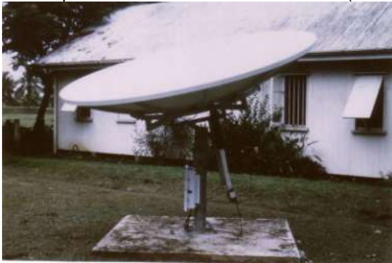
Figure: 5 Terminal at South Pacific Commission in Fiji, showing single axis motorised drive.
