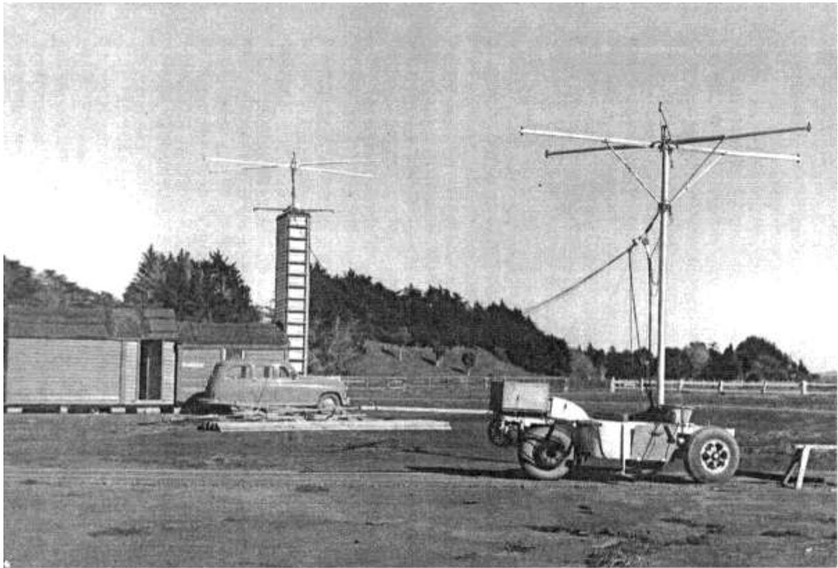
1953: MUCH WINDING – the first rotating interferometer for measuring bearing and elevation angles at Seagrove.
