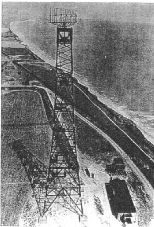
6. CHL on 185 ft tower and 20 ft gantry at Hopton
